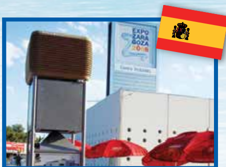
Bio-cooling tower at Zaragoza fair/expo (East coast of Spain)
