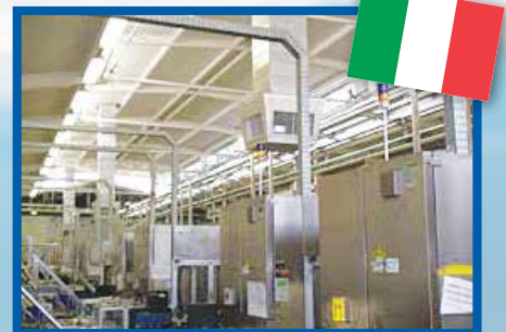
Granarolo factory (Italy)
